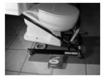
STEP 3 When ready to install same toilet or a new toilet, place new seal on cleaned floor flange, centered between flange bolts or on cleaned toilet horn.
