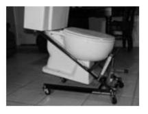
STEP 2 Use jack lever to raise toilet above old seal and flange bolts. Toilet can be rolled and safely held in desired area. Drain can be cleaned and cleared, sub floor and flange can be repaired, new floor can be installed, etc.
