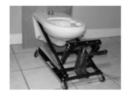
STEP 5 Install washers and nuts, snug by hand, release and remove jack. Tighten nuts to secure the seal and toilet to wall.
