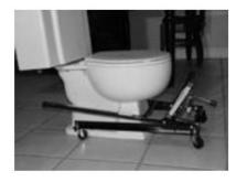
STEP 1 Close water valve, flush toilet, and disconnect supply line. Remove toilet bolt nuts and washers. Roll jack under toilet bowl.
