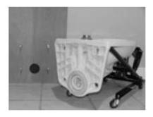
STEP 3 Back toilet away from wall and mounting bolts. Toilet can be rolled to desired area. With toilet safely held, the drain can be cleaned and cleared, old wax seal can be changed, etc.
