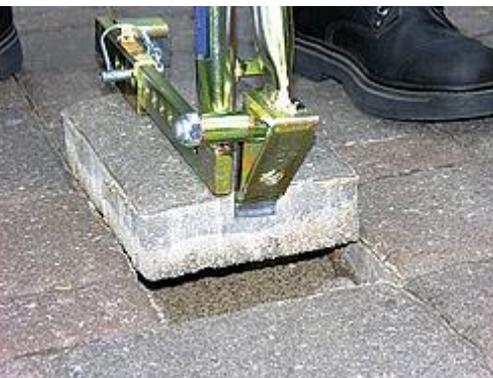
6. Continue removing pavers in the same fashion when the surrounding area is in need of repair. Replace with new paver(s) and sweep sand over the top. Take a piece of 2 x 4, place it over the new paver(s) and hammer with a mallet down the board's length, moving the 2 x 4 around the area. This will act as the compactor did during the initial installation. Fill the joints with sand.
