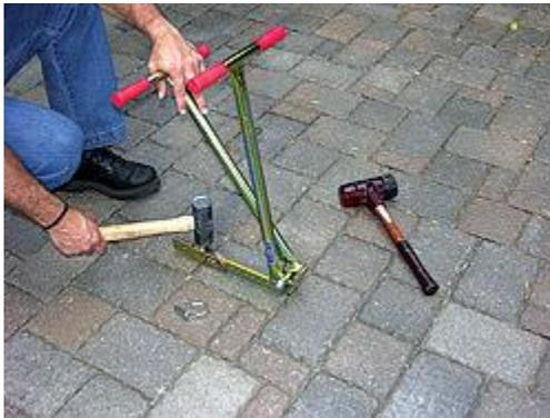
2. When it is time to set-up the PAVEREXTRACTOR, first remove the QUICKPIN. Then line up the teeth with the joint and hammer both ends down until the frame is tight to the top of the paver. It is critical that the teeth are down as far as possible.
