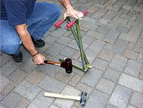
5. When the paver is difficult to extract, stop occasionally and tap the surrounding pavers. The process can be sped up by having one crew member work the PAVER EXTRACTOR while a second taps the surrounding pavers. Many times, there is so much interlock, the surrounding pavers are being lifted along with the paver being extracted.
